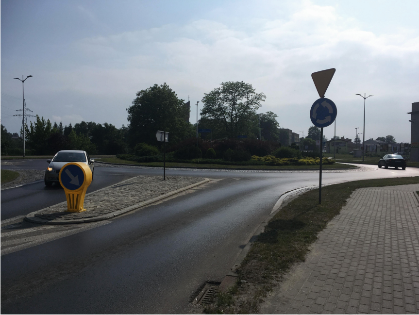
Fig. 2. An example of C-12 sign with A-7 sign on roundabout in Myszków, Poland
