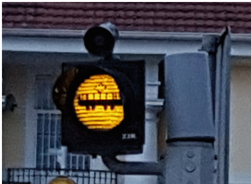
Fig. 10. Example of a traffic light used in Gdańsk for warning traffic lights located at pedestrian crossings leading through tram tracks
