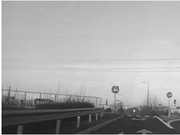
Fig. 12. Insufficient visibility caused by barriers securing pedestrian traffic
