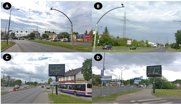
Fig. 1. ITS subsystem components in Bydgoszcz used to navigate drivers to alternative routes (A, B - ARCP cameras; C, D - city traffic status displays controlled by ITS)
