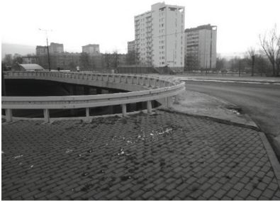
Fig. 8. Insufficient visibility caused by localization of energy-absorbing barriers
