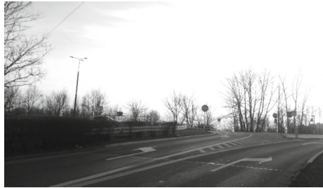
Fig. 13. Insufficient visibility caused by localization of energy-absorbing barriers
