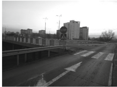
Fig. 9. Insufficient visibility caused by barriers securing pedestrian traffic
