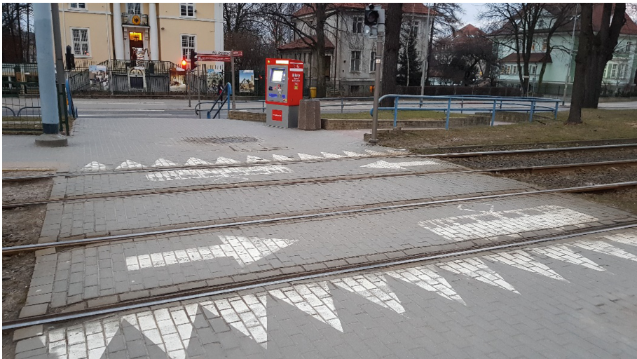
Fig. 6. Pictograms within pedestrian crossings leading through tram tracks within the analysed intersection
