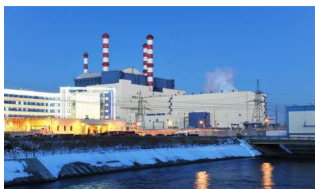
FIG. B-2. The BN-800 commercial fast reactor at the Beloyarsk NPP, Russian Federation, was connected to the grid in December 2015. (Photo: Rosenergoatom)
