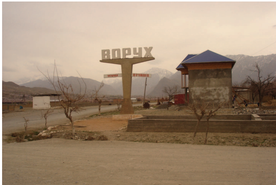
FIGURE 4. THE KYRGYZSTAN-TAJIKISTAN BORDER BETWEEN AK-SAI AND VORUKH IN MARCH 2008, SHOWING NEW CONSTRUCTION UNDERWAY
