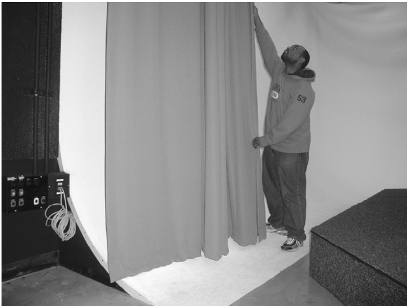
FIGURE 7.25 A sky cyclorama (skycyc) is a plain off-background that may be lit with a variety of different colors or patterns depending on the lighting instruments used. It also represents an infinite or nondescript background if that is called for in the set design. The cyc may be either a drape hung on a continuous rod to allow the drape to be moved and arranged as needed, or it may be hung as a hard cyc with both the corner and the section meeting the floor curved to add to the infinite background.
