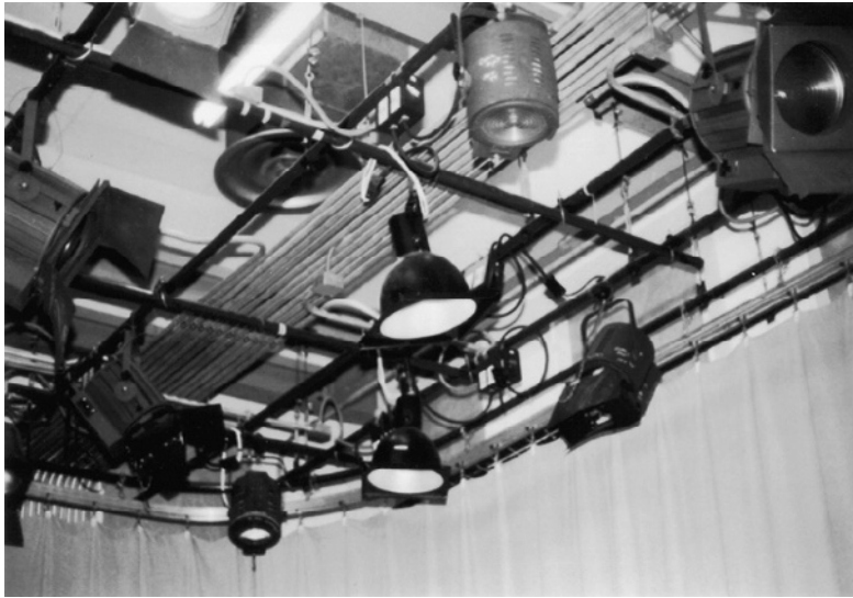
FIGURE 7.10 The lighting grid in a studio is constructed to support both the batten, which carries the power to the pigtails, and the lighting instruments. The grid must be high enough to allow wide-angle shots, but it also must allow for space above the grid to dissipate the heat generated by the lighting instruments.
