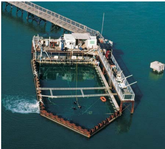
Excavation using a cofferdam: the wreck of the merchant brig designated YO 88 at Yorktown, Virginia, scuttled during the Revolutionary War.
