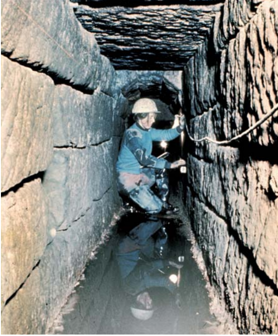
Examination of one of the Roman sewers still preserved beneath the city.
