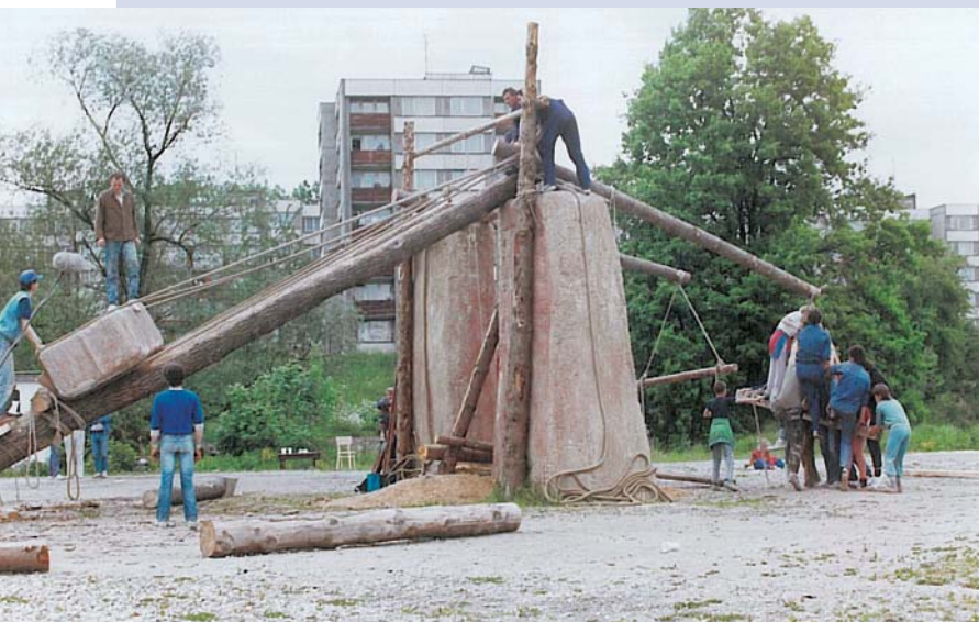
Reconstruction (above and below) of a possible method used to lift the lintel stones of the trilithons at Stonehenge.
