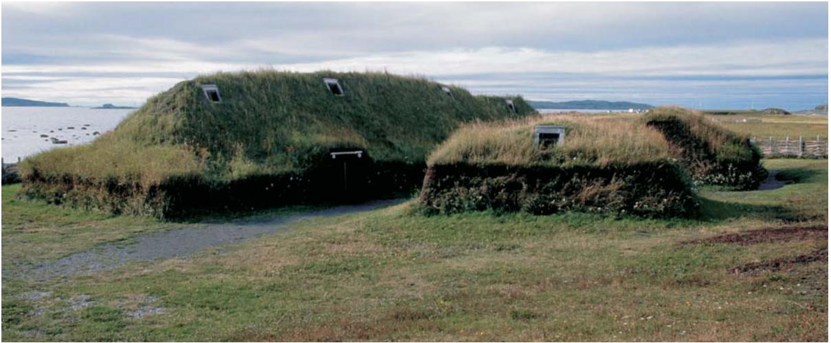
The low mounds at L'Anse aux Meadows turned out to be the remains of huts with walls of piled turf and roofs of turf supported by a wood frame – those seen here have been reconstructed for visitors. Lack of evidence for rebuilding indicates this was a short-lived settlement.
