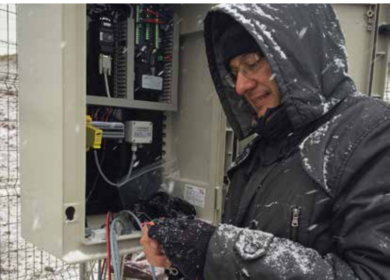
Installation works in Mingachevir water reservoir meteorological station
