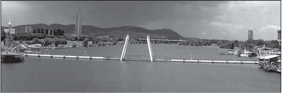
Figure 4.3 Floating pedestrian and bicycle bridge across the Danube tributary, Vienna, opens at mid-span for boat passage
