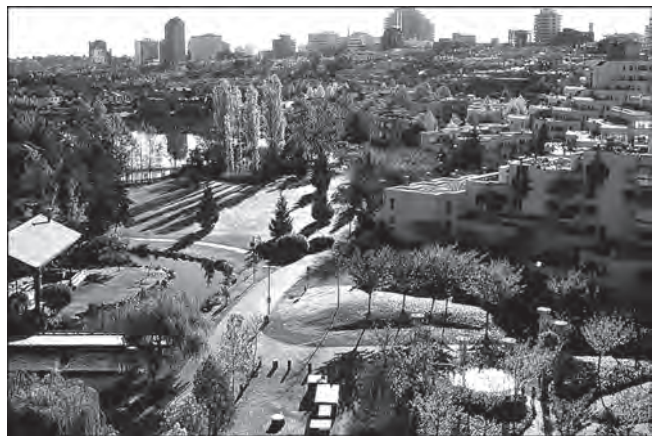
Figure 9.1 View of False Creek South, Vancouver, British Columbia – an area that would have been lost to freeway infrastructure and is now a walkable neighbourhood
